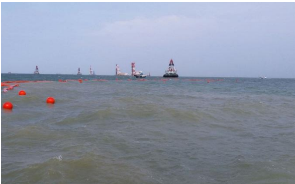
Photo 3: Sea condition inside the silt curtain during the pilot test
