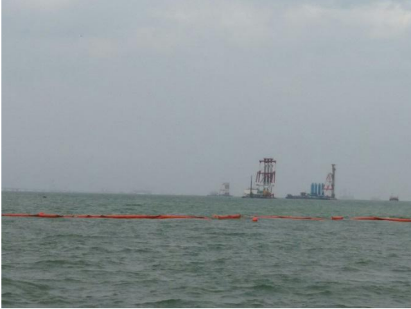
Photo 1: Deployed section of silt curtain for pilot test
